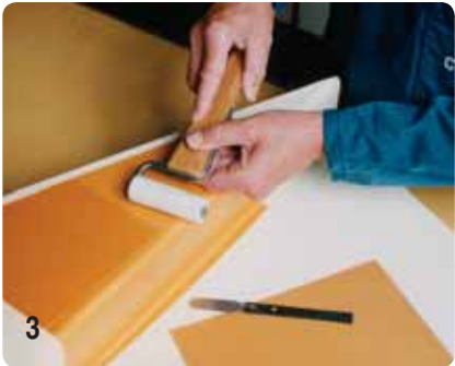
Roll to extrude air bubbles for a flat, even surface.
