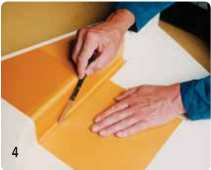
4 Accurately fitting subsequent pieces.
