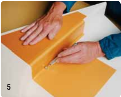
5 Consolidation of corners using filletting tools.
